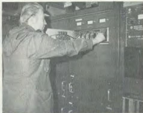
...Mraz inspecting printed circuit boards in the AC control...
