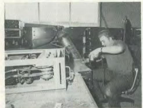
.... Roy Mraz working on assembly of an SCR module in service building D-0...
