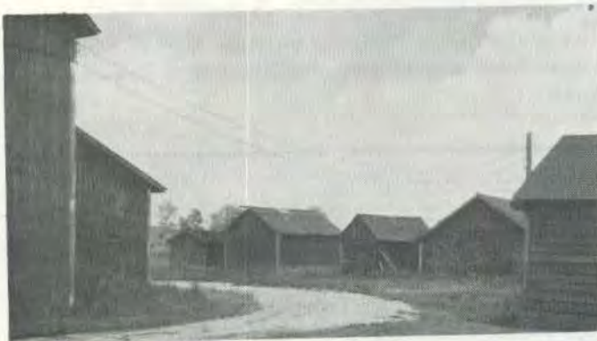
...The outbuildings on the former Schimelpfenig Farm will be removed during November...
