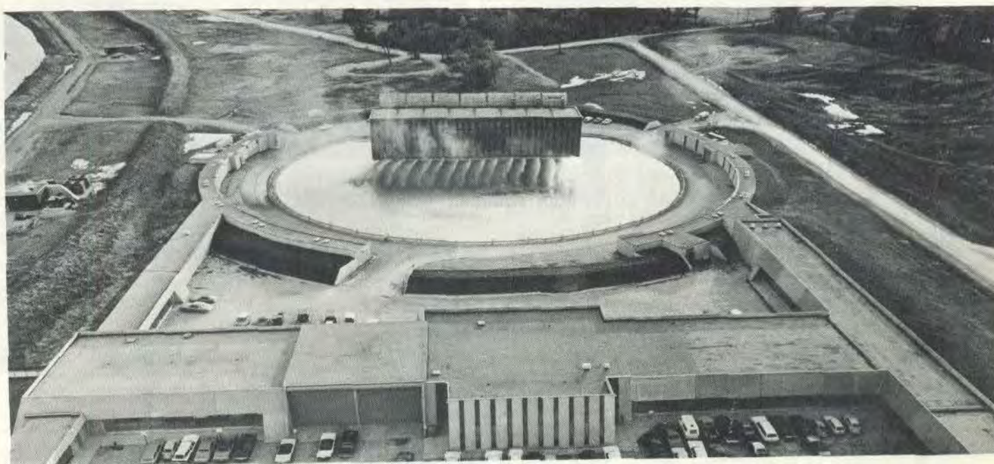
...NAL Booster accelerator as seen recently from the 15th floor of the Central Laboratory building by photographer Tony Frelo. Curving at upper left is Main Ring berm; Linear accelerator is at right; Cross Gallery horizontally at bottom...
