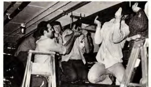
...RF crew installs bus bar in Booster Accelerator...
