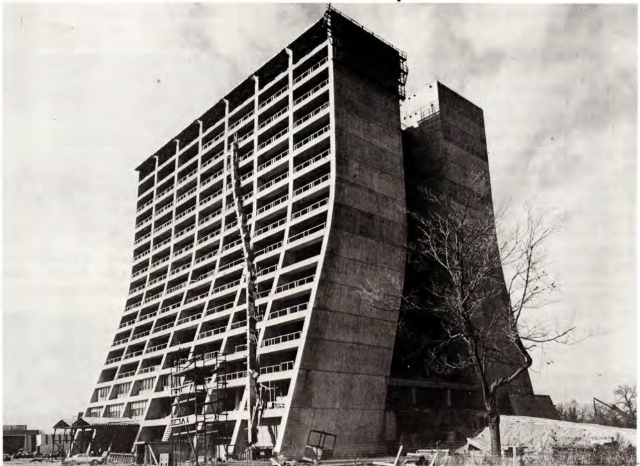
...The top floor of NAL's Central Laboratory Building is now being poured. The building will be ready for occupancy some time after March, 1973. It will house many of the functions of the Laboratory including all of those now located in the NAL Village...
