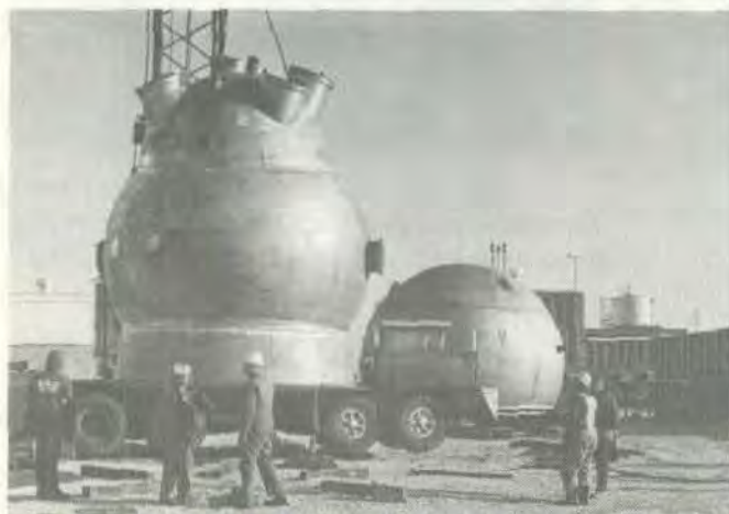
....The 15 foot bubble chamber arrives "home" after a temporary stop in The Village, following its arrival on October 25. Hemisphere on the ground is the upper portion of the vacuum tank which surrounds the chamber....
