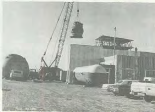
....The 15 foot bubble chamber arrives "home" after a temporary stop in The Village, following its arrival on October 25. Hemisphere on the ground is the upper portion of the vacuum tank which surrounds the chamber....
