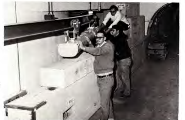
...Tony Rader (L), Ron Norton, Jerry Czop move Doubler prototype into place in Main Ring tunnel...
