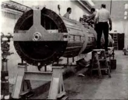
Linac tanks were built in the NAL Village (L), then moved (above) to permanent location.
