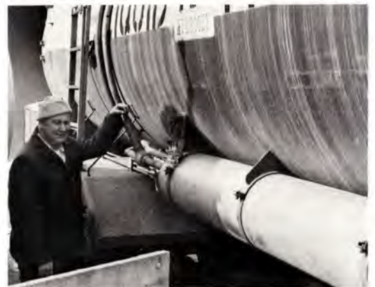
...Paul Thorkelson at controls of liquid neon/deuterium storage tank he built with Larry Biggam...
