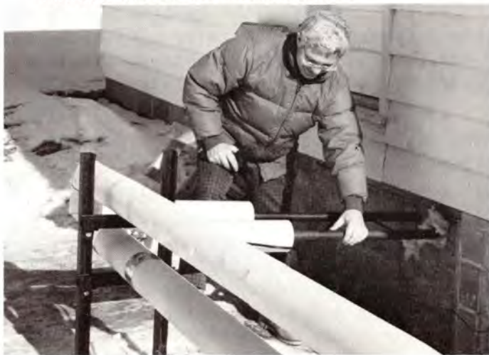
...Heat in water from solar collector panels enters heating system of house...
