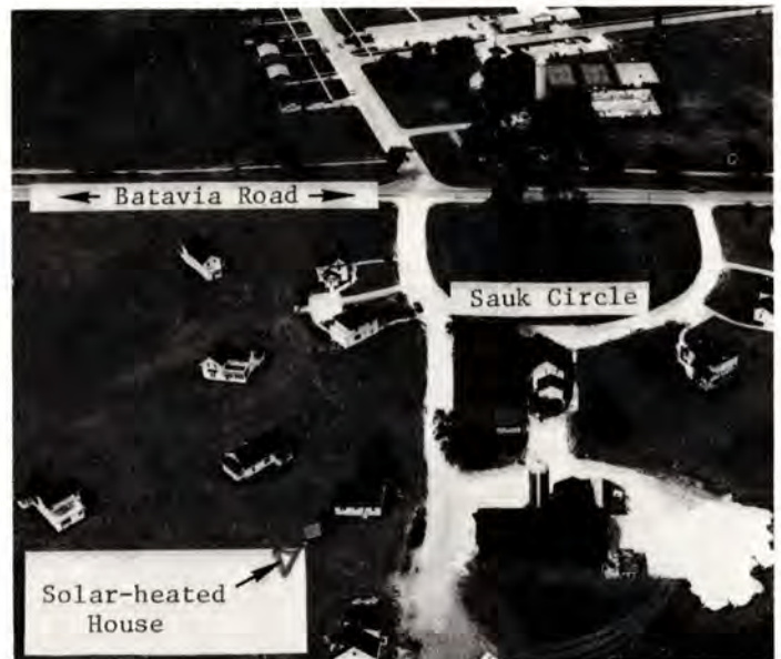
...Solar Energy House at Fermilab on Sauk Circle...
