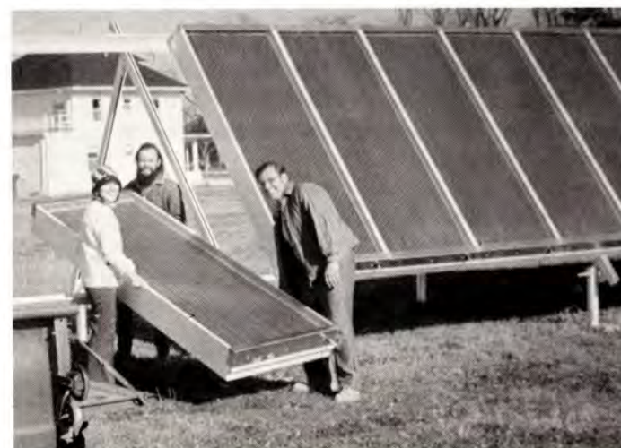
...J. Sutcliffe, S. Bastian, J. Carson raise panels to outside frame...
