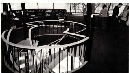
... Two interlaced spiral staircases lead up to control center...
