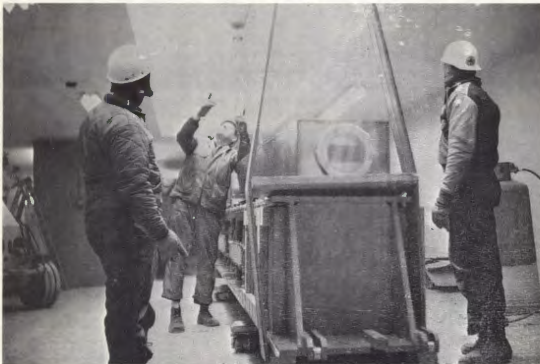
Putting the first Booster module in place....
