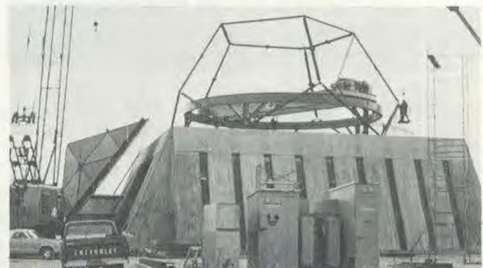
4) Steel frame was erected on top of Bldg. A as a base for the 3.8 ton completed sections which were raised by cables attached to cranes..
