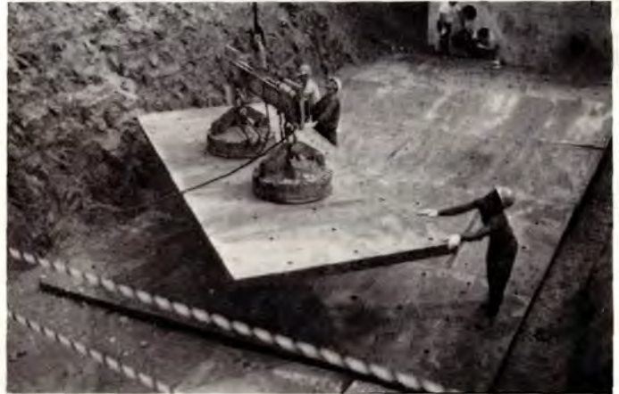
...Unloading armor plate at Fermilab...
