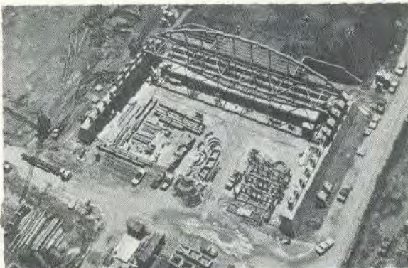
...Main building of Meson Laboratory now under construction...
