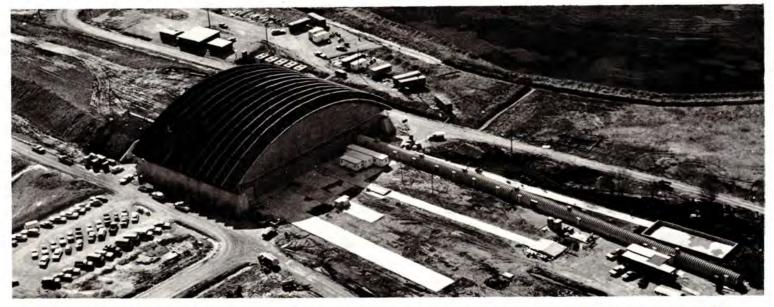
...An aerial view of the Detector Building and some of the experimental lines of the NAL Meson Area. Since the photo was taken in April, 1973, enclosures, the same as over the M6 Line, have been completed over the M1 Line and the M2 Line (the two lower rectangles extending from the building). Main accelerator is to the left (southwest) of the building...
