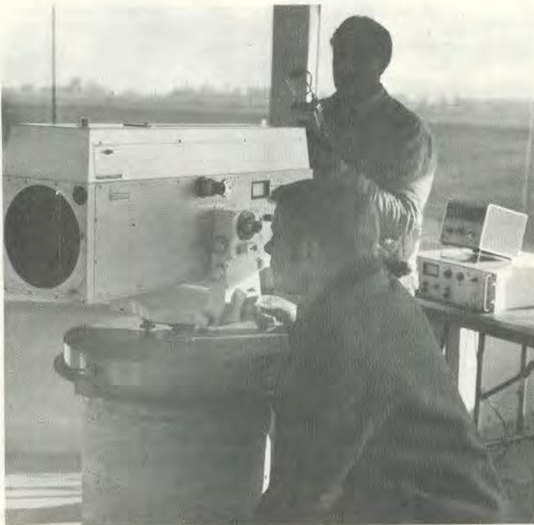
DUSAFers Gerald Edler (right) and John Chism operate distance-measuring laser in The Gazebo, survey tower in center of Main Accelerator ring.
