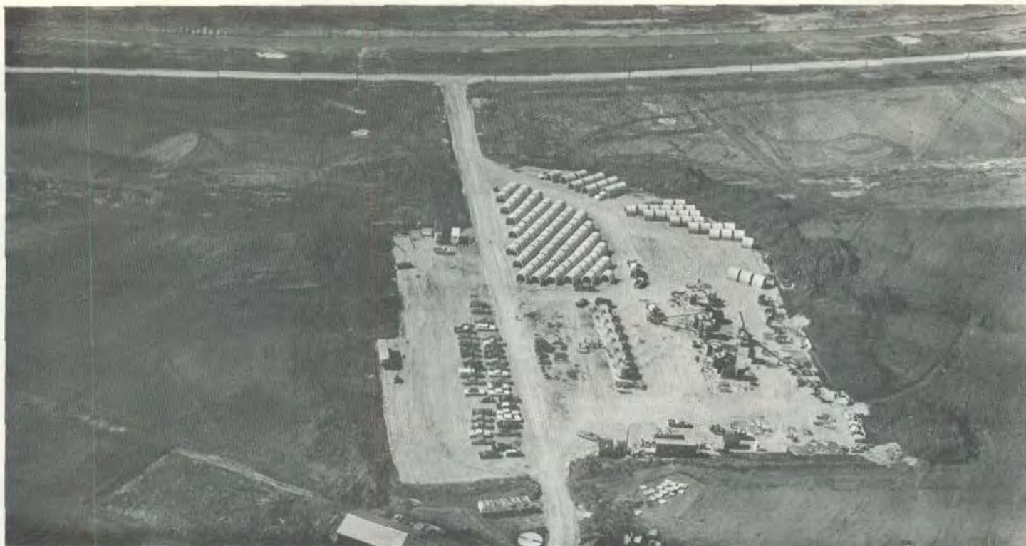
MAIN RING SECTIONS START HERE: An aerial view of Main Ring enclosure concrete sections in the pre-cast yard near Eola road. The sections are poured and cured here and then trucked to the sites excavated for the Main Ring---a four-mile-in-circumference enclosure that will be the main component in the NAL accelerator system. (Photo by Tony Frelø)
