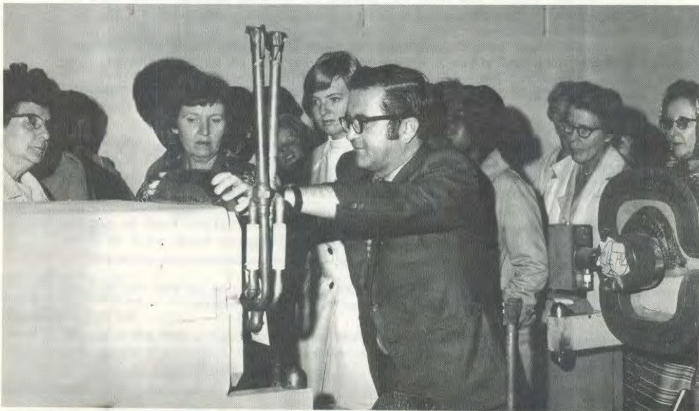
....An orientation tour for NAL's female personnel to brief them on construction progress and plans for the permanent site was held Monday, September 14. Thirty-seven ladies joined the tour, arranged by Doris Ferrell, which included a one-hour visit to the Linac, Booster and Main-Ring areas. Donald Getz, Assistant Laboratory Director, (center above) led the tour. The above photo was taken during the tour....
