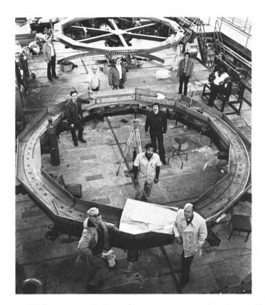
...Chicago cyclotron's upper cryostatic coil assembly in the background, already wound and welded shut. Lower assembly in the foreground is waiting to be wound. Photograph taken in the Meson Detector Building. Clockwise, outside lower assembly are John Rauch, Ed Tilles, Bob Kephart, Steve Dochwat, Clarence Rodgers, Joe Heim and Jim Michelassi. Clockwise inside the lower assembly are Richard Applegate, Gary Wisniewski and Chet Shaw...
