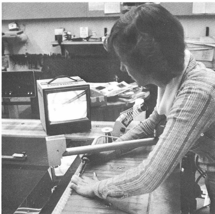
...Mary Rothengass looks at the screen to make sure she's soldering a wire in the correct position...
