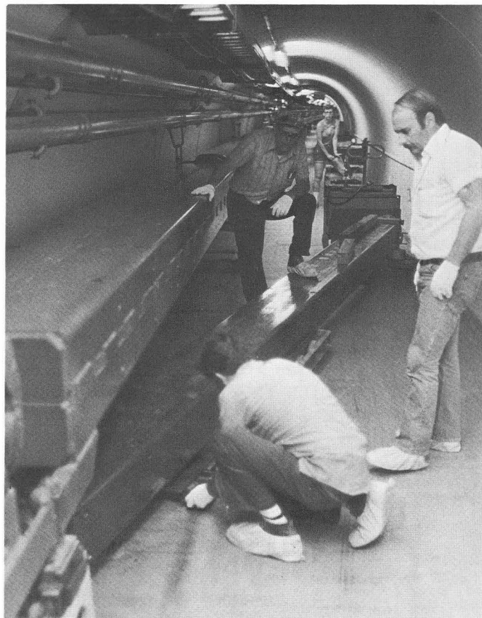
...Putting a superconducting dipole magnet into place just below the string of conventional magnets in the Main Ring tunnel...
