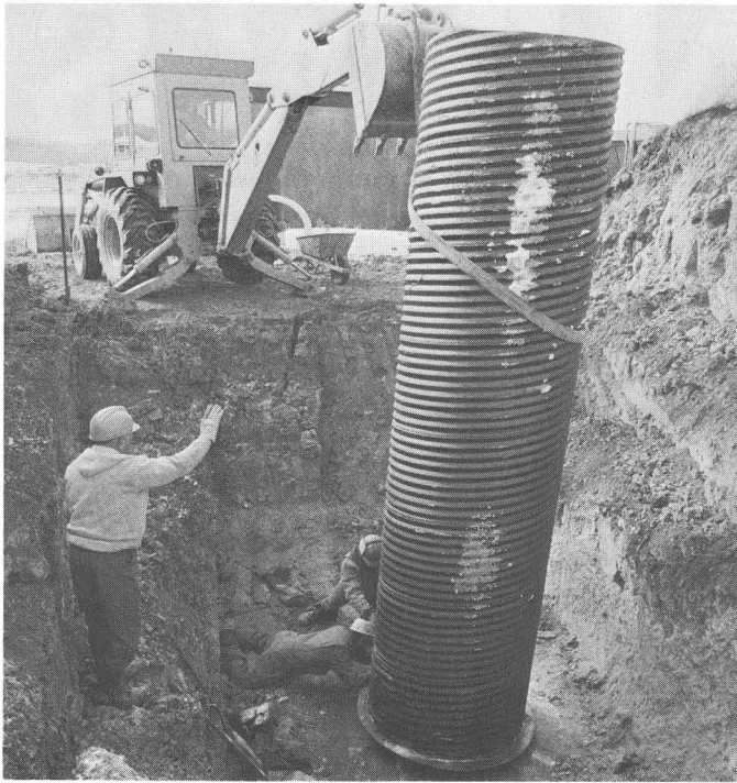
...Workmen install penetration tube on top of the Main Ring tunnel...
