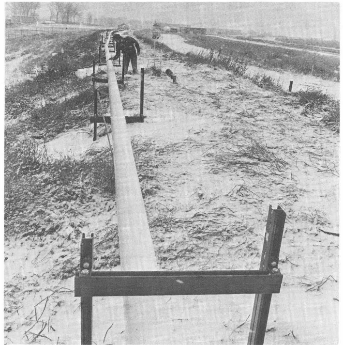
...Paul D. Brindza, engineering physicist with the Cryogenics Systems Group, inspects the recently completed helium transfer line that runs from A-1 to A-2 on the berm of the Main Ring. This view is toward A-2. Liquid helium is made from gaseous helium at A-1 in quantities of 100 liters each hour. The liquid helium is then pumped through the transfer line to the A-2 refrigerator. There the helium is consumed and runs A-2 as a satellite refrigerator. In the background (just above Brindza's head) is a moveable tent in which sections of the line are welded together. Brindza expects the line to be operational sometime near the end of February. Eventually the transfer line will run the full four miles around the Main Ring...
