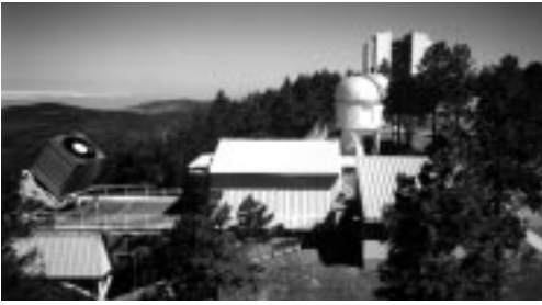
Apache Point Observatory in the Sacramento Mountains of New Mexico. The Sloan Digital Sky Survey's 2.5-meter telescope is on the left. The monitor telescope, used for calibrations, is inside the small domed structure.
