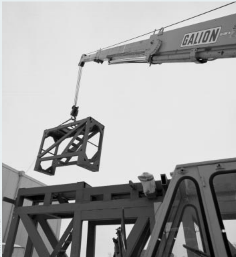
The crane truck carefully lowers a side section into place atop the 25-ton base.
