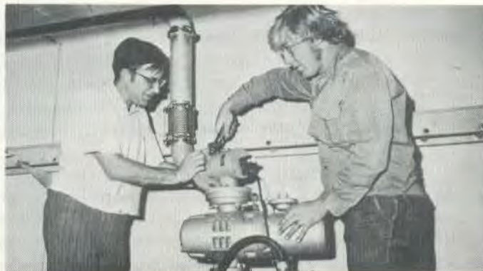
...Jerry Czop and Frank Juravic work on a vacuum pump in Enclosure H...
