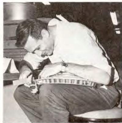
...John Zuk assembling old screen capacitor...
