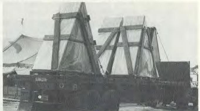
2) Crew of 5 men assembled 120 panels at rate of 6 per day. Panels were moved from the assembly area to the bubble chamber area by truck..
