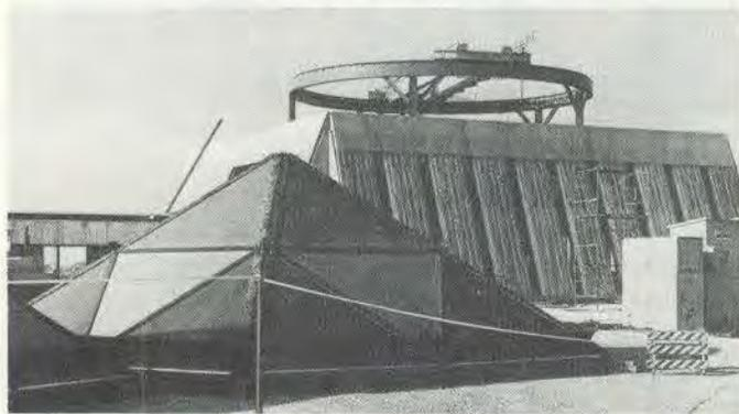
3) Next stages of assembly took place adjacent to Building A, shown in background. Circular crane now used in assembly work extended over top of building..
