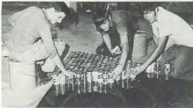
1) Each panel, a triangular "sandwich" of 2 slices of polyester-reinforced fiber-glass spread with a coating of epoxy, was pressed together by sand bags overnight..
