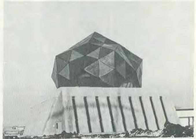
...Geodesic dome atop Building A of the NAL Neutrino Laboratory, constructed of triangular sandwich panels containing discarded beverage cans donated by the public...
