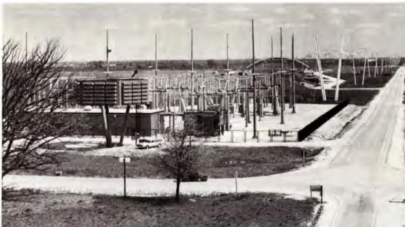
...Fermilab Master Substation. Foreground, left, capacitor tree to level peak demands from accelerator at 500 BeV...
