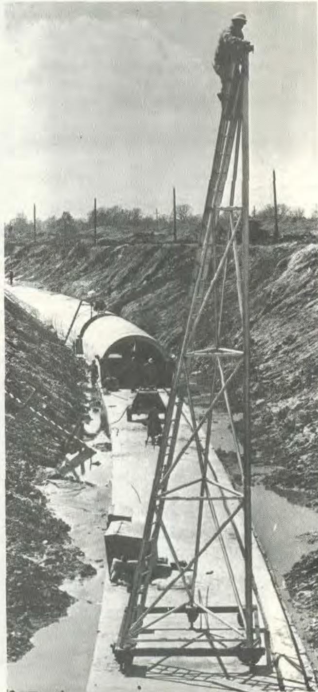
A workman on tower makes target adjustment for laser beam, used as a modern surveying device in construction of NAL's Main Accelerator enclosure. (Chicago Sun Times photo)
