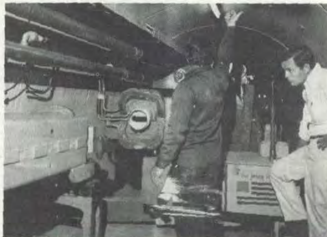
...(L to R) Tony Winchester, George Hill install a replacement magnet in the Main Ring Tunnel...
