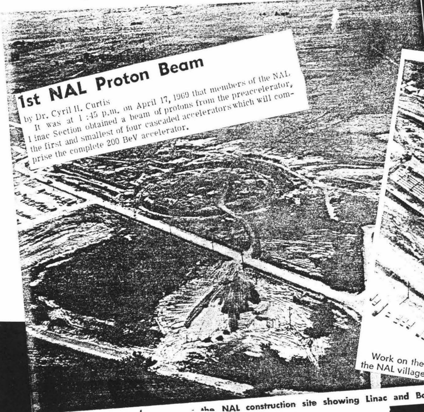
A late August aerial view of the NAL construction site showing Linac and Booster enclosures.
