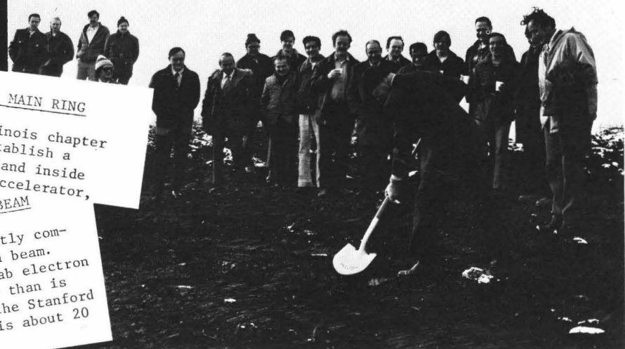
...Fermilab Director R. Wilson's spade signals start of Internal Target Addition...
