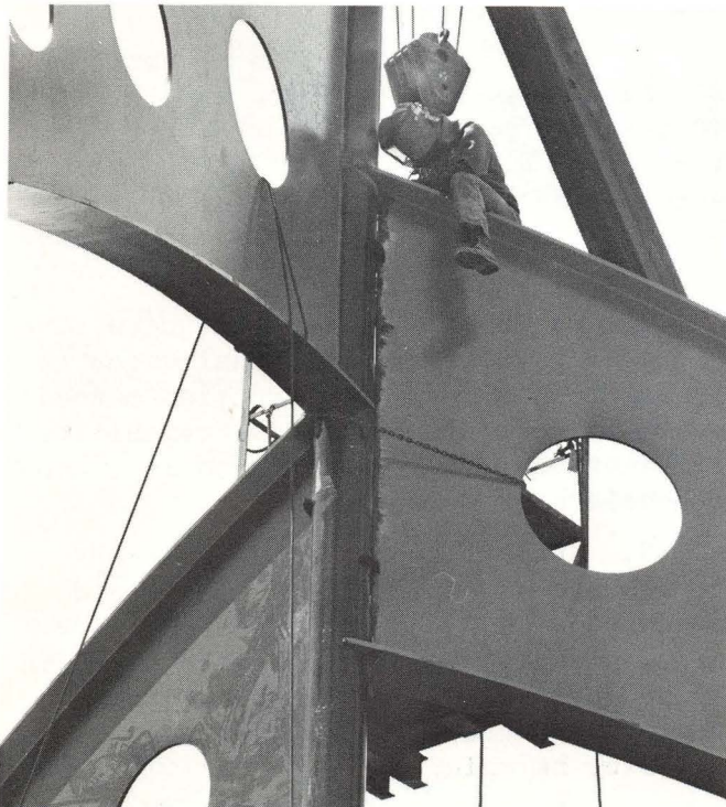
...Welder joins three "Legs" to pipe...
