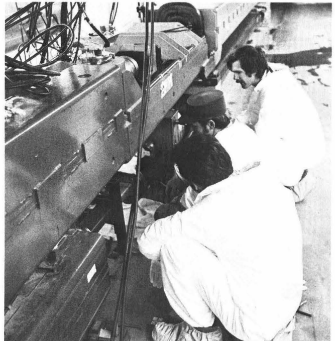
...Technicians install superconducting magnets in Main Ring for tests and evaluation...
