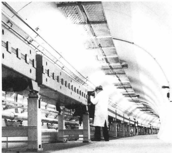
...Inside the CERN SPS tunnel...
