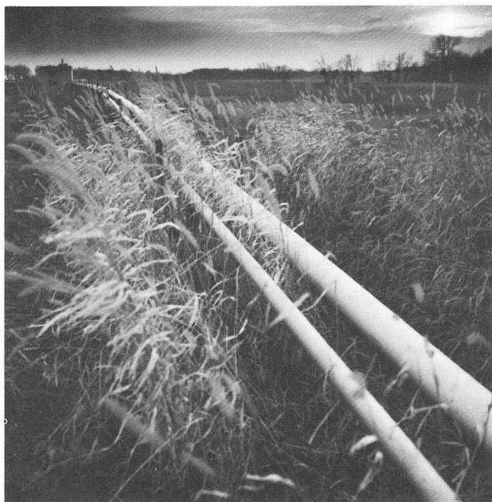
Closeup of transfer and high pressure helium line on top of the Main-Ring berm (see aerial photograph on preceding page).
