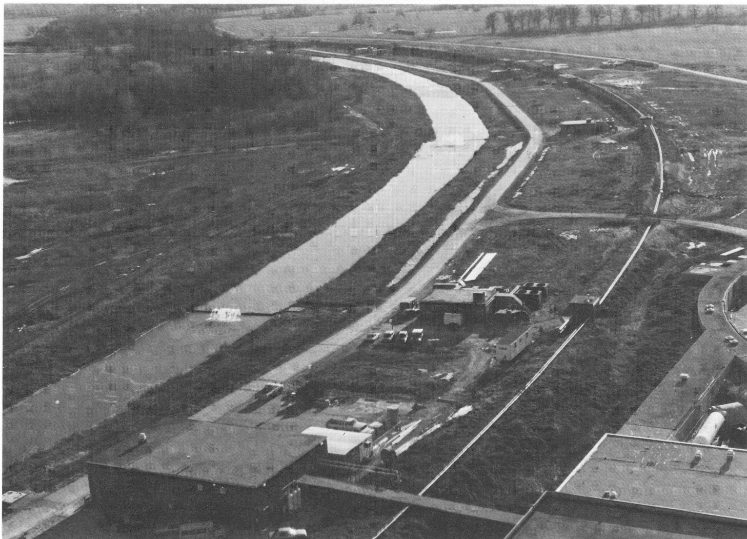
Aerial view of the Main Ring near A0 showing completed section of transfer and high pressure helium line.
