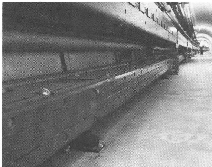
Energy Saver magnets and helium line installed under conventional magnets in Main-Ring tunnel.
