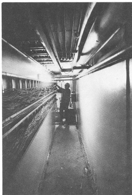
A contract electrician installs control cable at E4.
