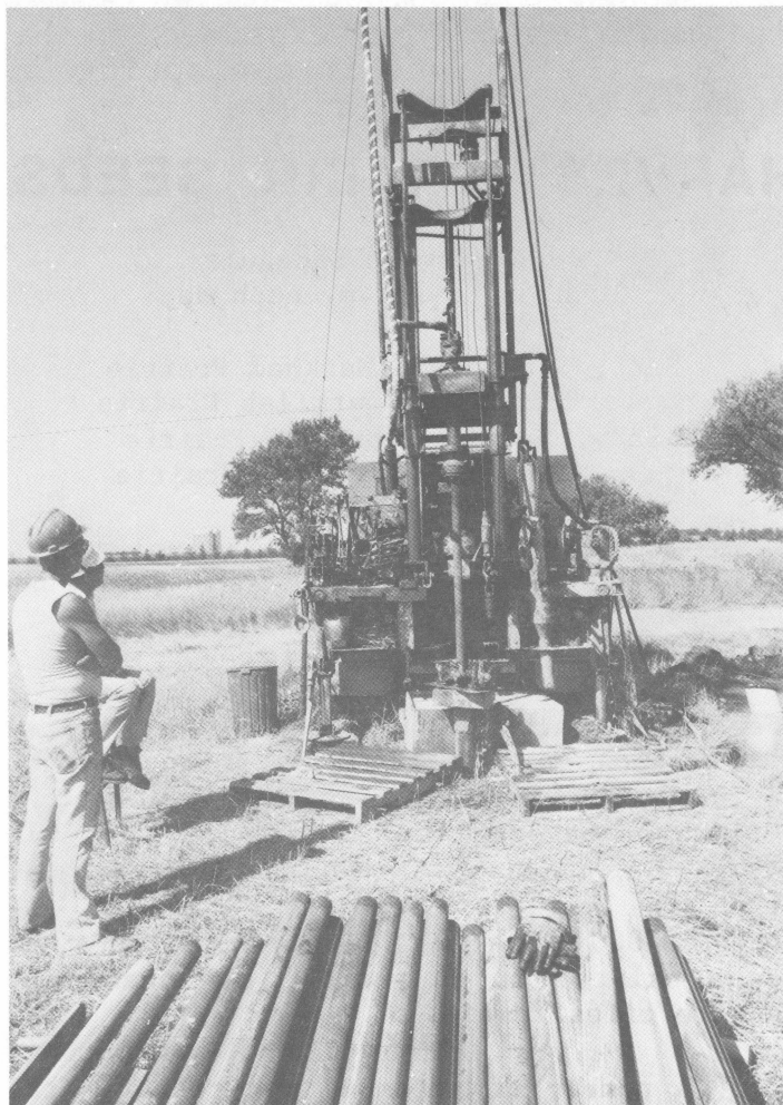
Drilling rig boring a 500-ft deep hole near the corner of Batavia and Eola Roads on the Fermilab site.
