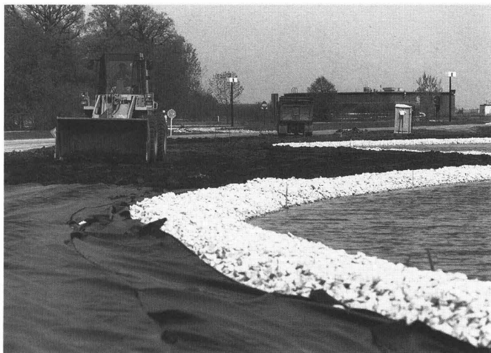
Workers put the final touches on the Swan Lake project.
