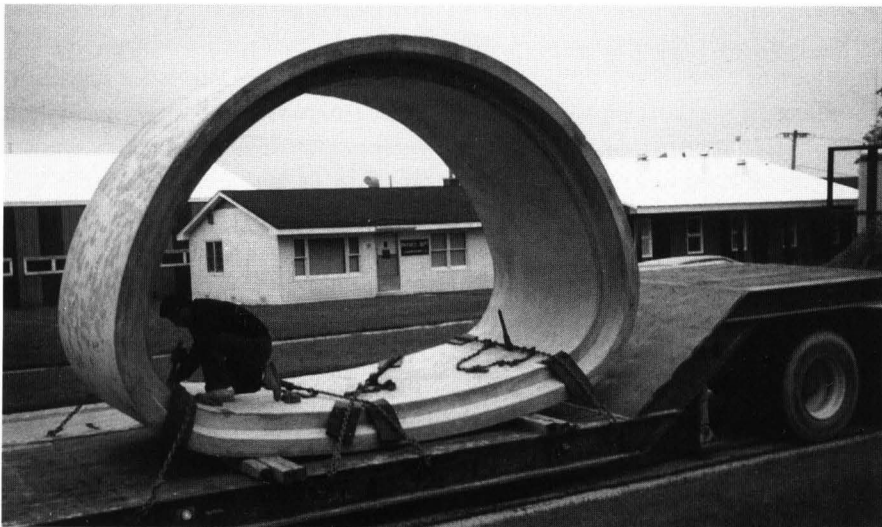
A worker prepares to unload a section of the prefabricated tornado shelter. Five sections, each 25 x 15 feet and weighing 17 tons, were installed next to Lab 8.
