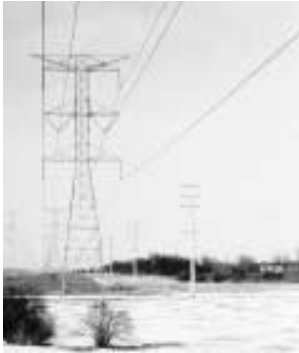
A view of the Lab's eastern border with the Summerlakes subdivision in Warrenville on the right.
