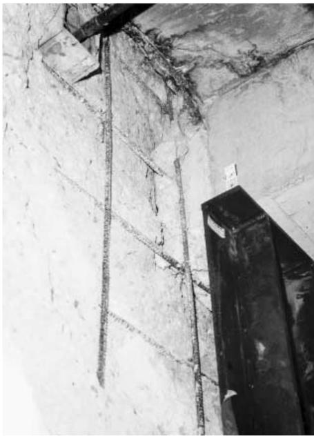
Seasonal stresses on structural beams have exposed these steel support rods in the concrete.
