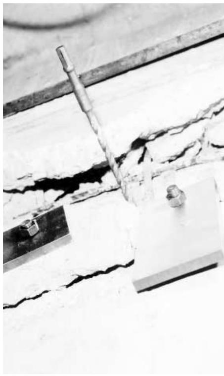
Reinforcing plates hold loose pieces of concrete in place.
