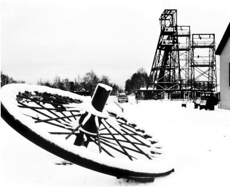
Wheels like this one in the headframe (background) raise and lower the elevator that carries tourists and workers down into the historic Soudan mine.
