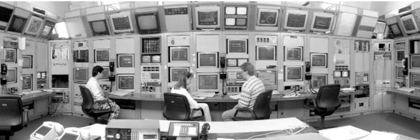
The Main Control Room contains readouts on more than 100,000 channels of information, with controls for 44,000 devices in the Fermilab accelerator complex.
