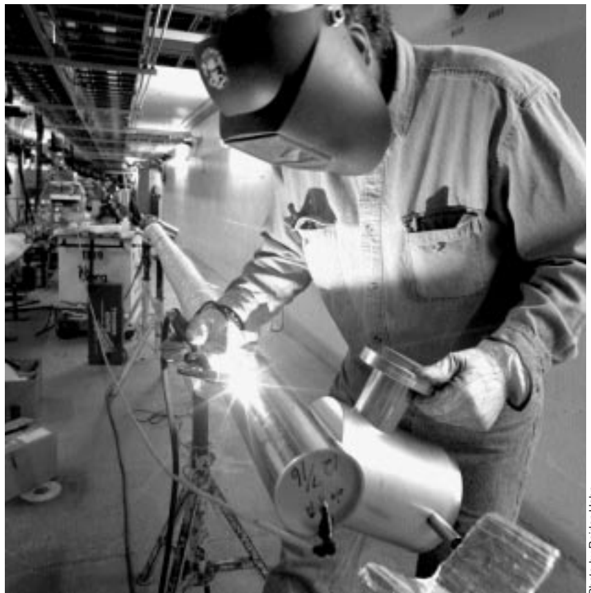
The Recycler contains two miles of beam pipes. Welding the vacuum tubes created airtight connections.
