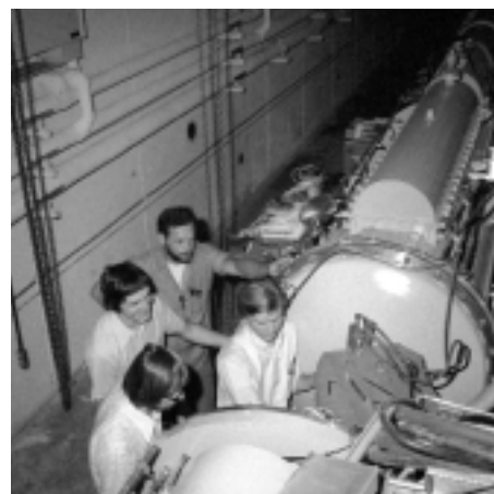
Scientists had to install a magnet in the beamline of the already existing linear accelerator to extract proton beams and direct them to the neutron production target.
