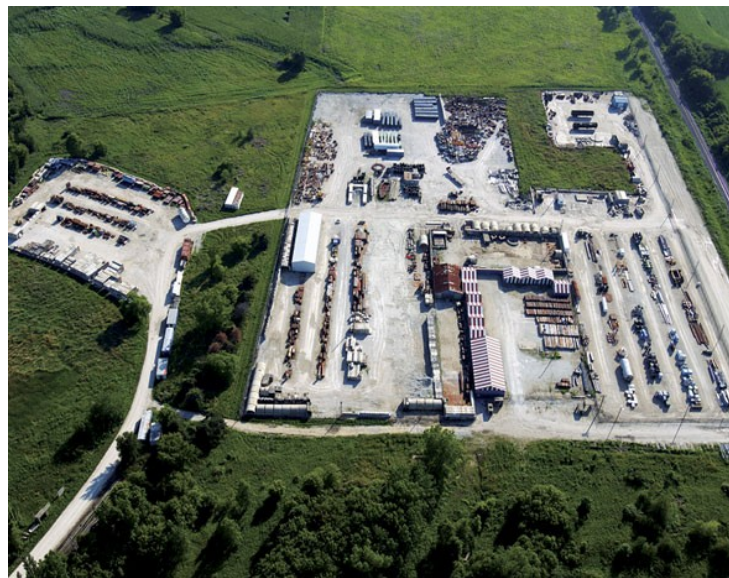
Figure 4. An aerial view of the Fermilab “boneyard,” with the Burlington RR visible on the right.
